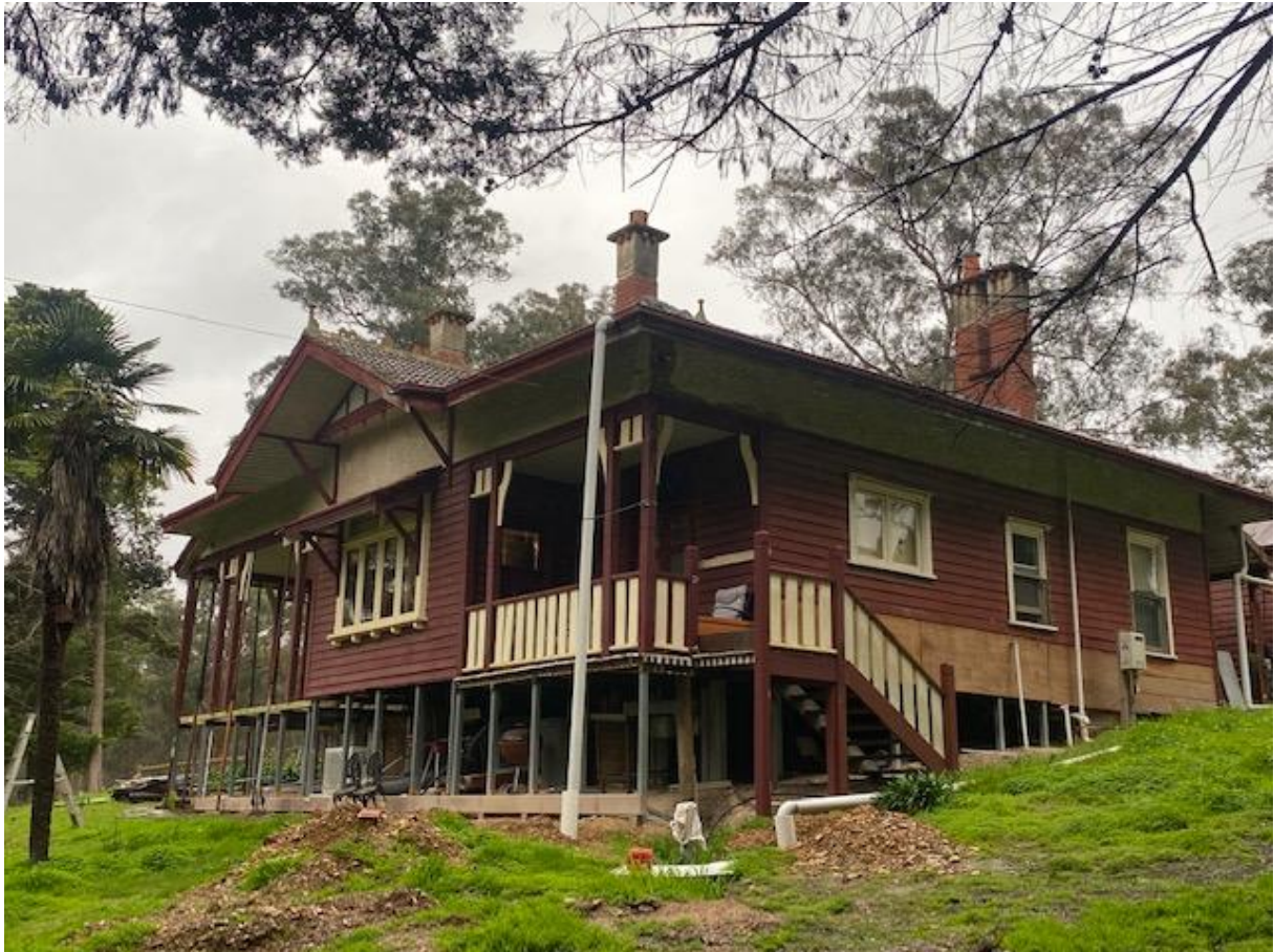
Figure 6. The southwest corner northwest elevation of the house. Note the projecting gabled bay, roughcast render panel beneath the eaves line, window awning and decorative timber fretwork to the verandah. (Source: Nillumbik Shire Council, July 2021)
