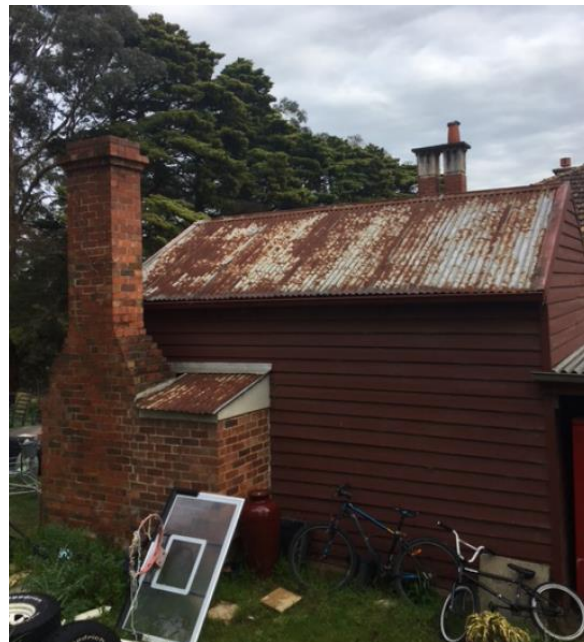
Figure 7. Weatherboard outbuilding located to the southeast of the house. Note the walls have been recently reclad, the window replaced and brickwork appears to have been added to the base of the chimney. (Source: Property owner)
