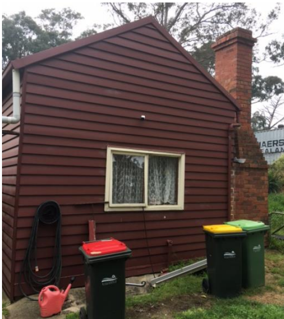
Figure 7. Weatherboard outbuilding located to the southeast of the house. Note the walls have been recently reclad, the window replaced and brickwork appears to have been added to the base of the chimney. (Source: Property owner)
