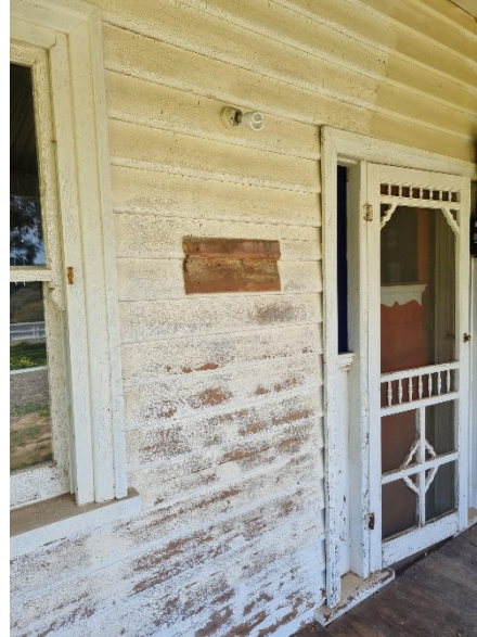
Figure 14. Decorative timber fly screen door with half glazed front door behind. Note the unpainted panel on the wall where an original name plate would have been located. (Source: Nillumbik Shire Council, photograph of owner)
