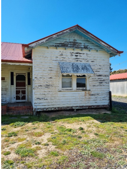
Figure 13. Projecting front room with decorative gable end above a pair of timber double hung sash windows with a timber window hood supported by brackets with scalloped trim. (Source: Nillumbik Shire Council, photograph of owner)
