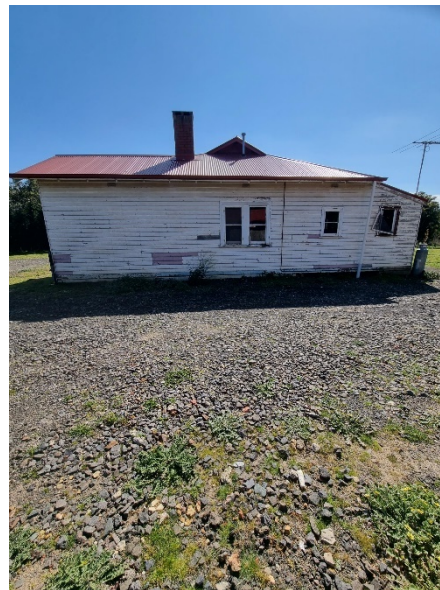
Figure 16. South elevation showing Dutch gable end, red brick chimney, pair of double-hung sash windows. (Source: Nillumbik Shire Council, photograph of owner)
