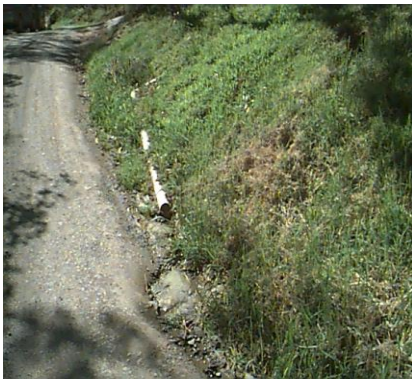
Figure 1: Greywater discharge to street culvert in Doleen Road, North Warrandyte
