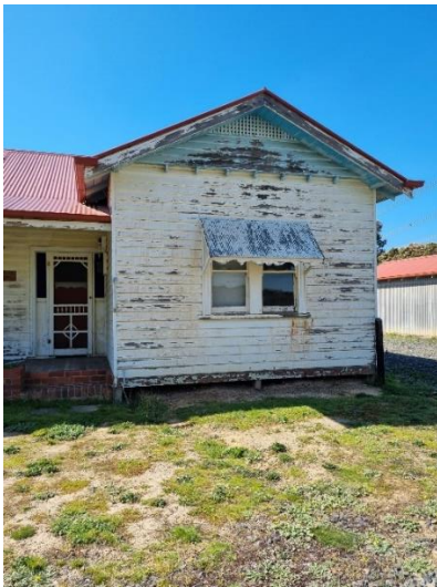
Figure 8 Projecting front room with decorative gable end above a pair of timber double-hung sash windows with a timber window hood supported by brackets and with scalloped trim. (Source: Nillumbik Shire Council, photograph of Owner)
