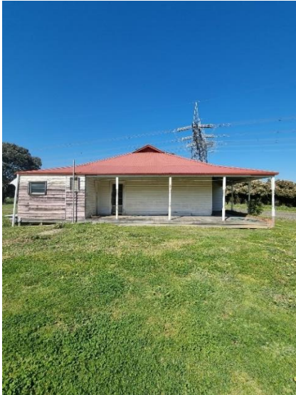
Figure 10 North elevation showing the original return verandah with turned timber posts and dutch gable end. (Source: Nillumbik Shire Council, photograph of Owner)
