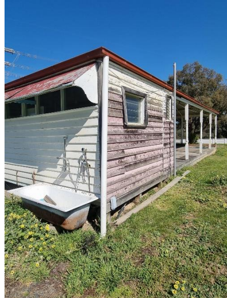
Figure 13 Northeast corner of the house showing the enclosed verandah which is evident in the 1936 photograph (Figure 1). Note the extant early window hood that runs the length of the east elevation. (Source: Nillumbik Shire Council, photograph of Owner)
