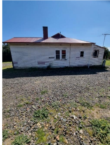
Figure 11 South elevation showing the house's original dutch gable end, red brick chimney and pair of double-hung sash windows. (Source: Nillumbik Shire Council, photograph of Owner)
