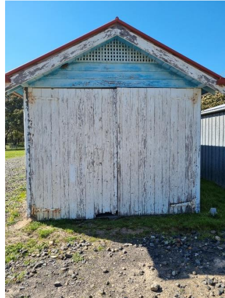
Figure 15 Early timber garage which is evident in the 1936 photograph with lattice gable end detail that matches the house. The timber doors appear to retain their original hinges. (Source: Nillumbik Shire Council, photograph of Owner)
