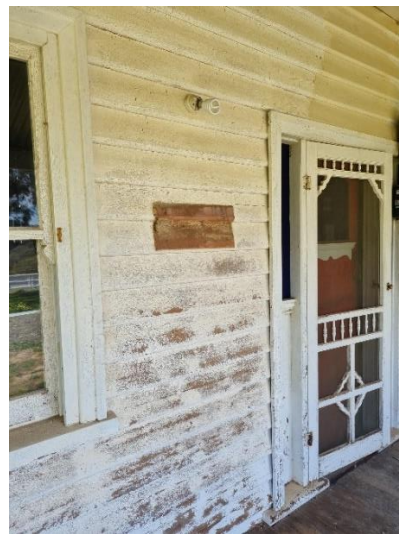
Figure 9 The original decorative half-glazed front door is visible behind the fly-screen door behind. Note the unpainted panel on the wall where the name plate would have been located. (Source: Nillumbik Shire Council, photograph of Owner)
