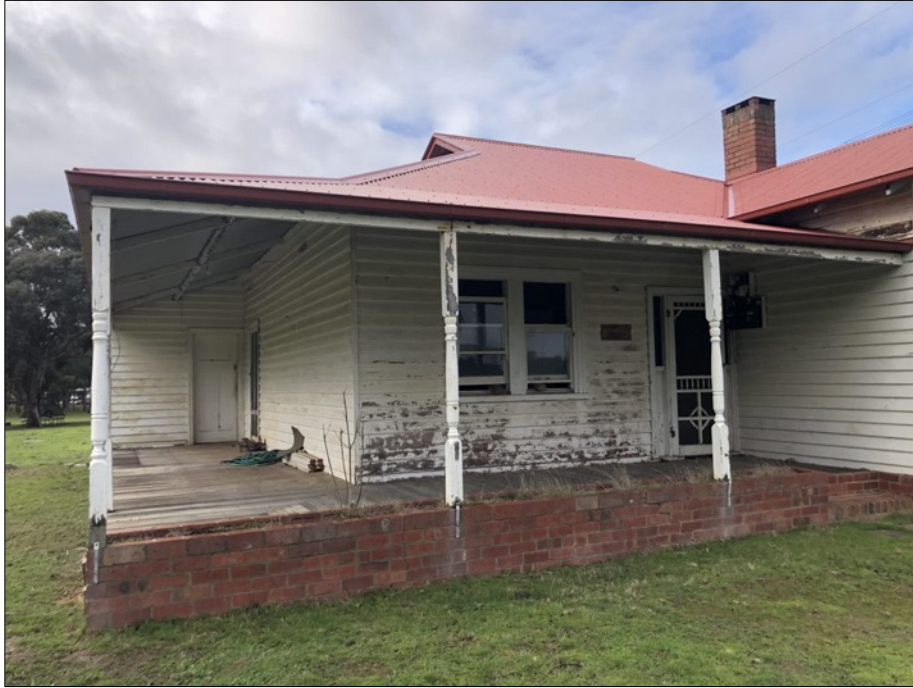
Figure 8 A brick planter box and steps have been introduced to the front verandah, truncating the timber verandah floorboards on this elevation.
