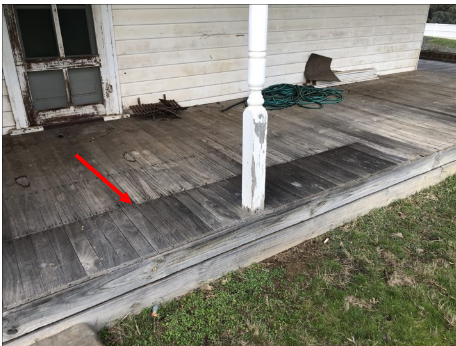
Figure 7 The repairwork/part replacement made to the verandah floorboards is indicated by the red arrow.
