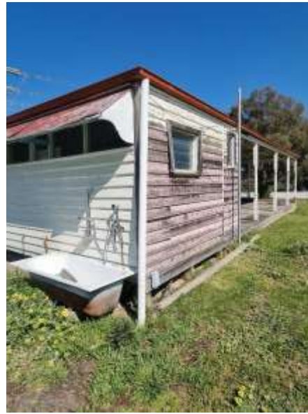
Figure 18. Northeast corner of the house showing the enclosed verandah. Note the extant early window hood that runs the length of the east elevation. (Source: Nillumbik Shire Council, photograph of owner)
