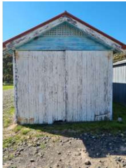
Figure 20. Timber garage with lattice gable end detail that matches the house. The timber doors retain their original hinges. (Source: Nillumbik Shire Council, photograph of owner)
